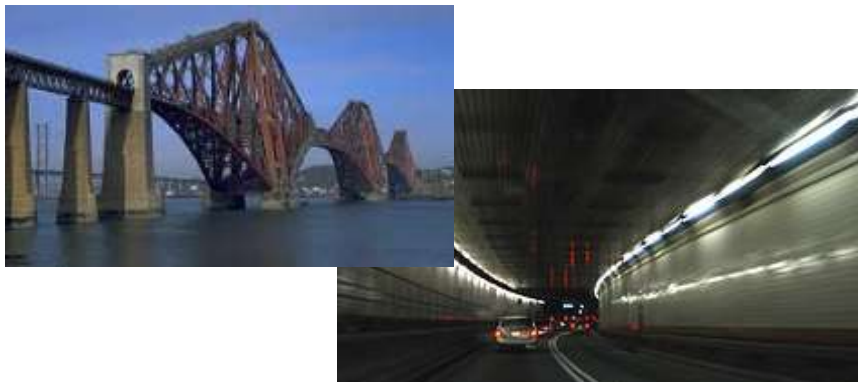
Bridge/Tunnel Safety Monitoring
